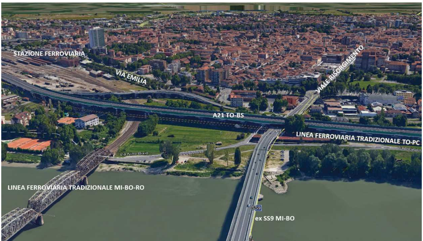
Fig. 3.3 Infrastructures, Po river and city of Piacenza. Processing from a bird's eye view of Google Earth.
