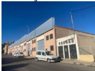
Buildings to be removed
