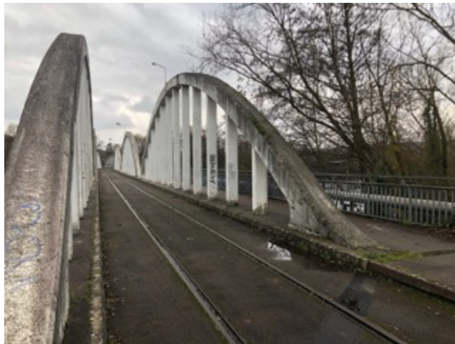
Bow String Bridge in Pompey, France
