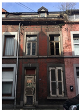
A. State of ruin, safety danger
